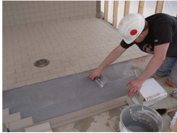
Installer trowels on Thinset® Adhesive adjacent to bonded, pre-spaced tiles.
